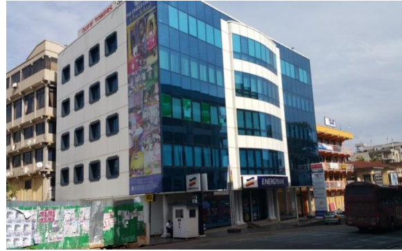
Fig. 12 Extensive use of glass and alucoboard in "Dufie Towers" Source: Authors, 2016
