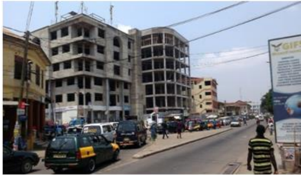
Fig. 3. Two multi structures under gentrification opposite the Akyampemhene's palace along the Guggisberg road Source: Authors, 2016
