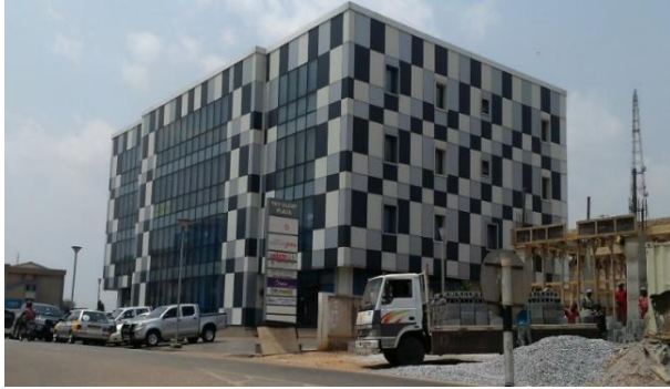
Fig. 12 Extensive use of glass and alucoboard in "The Glory Plaza" Source: Authors, 2016
