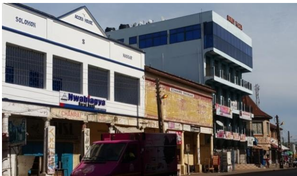
Fig. 5. The Accra house and Edward Nassar building not gentrified along Guggisberg road; Source: Authors, 2016
