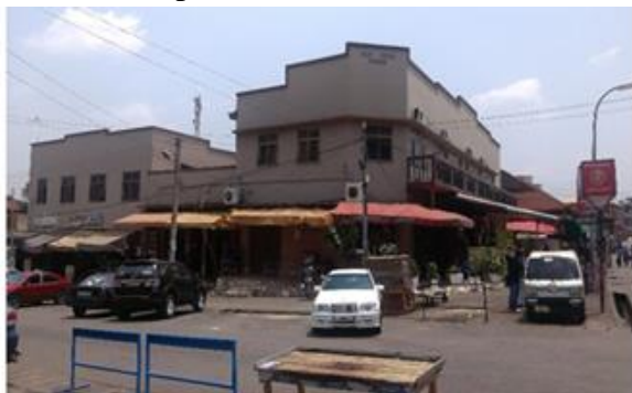
Fig. 10. Adumhene's Palace being conserved Source: Authors, 2016
