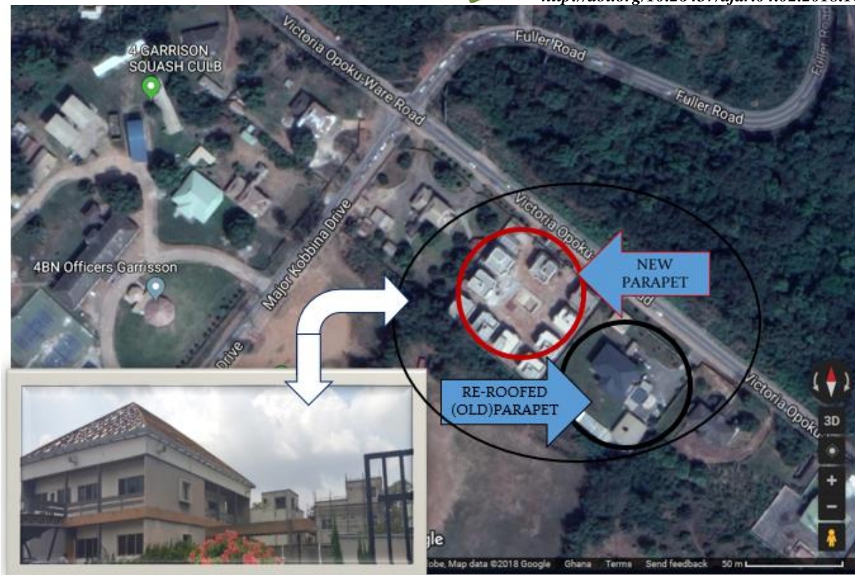
Fig. 3. A parapet roof completed in 1976 being re-roofed and a new concrete parapet roof building on the next plot of land along Victoria Opoku-Ware Road. Source: (inset) Authors, 2016; Google maps, 2018.
