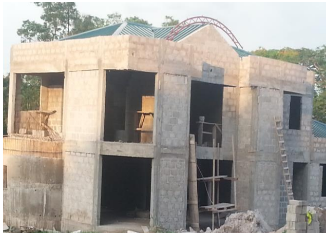
Fig. 5. New Concrete Parapet Roofs. Source: Authors, 2016
